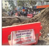
Site Visit to Underground Gutter Construction, Nashik
